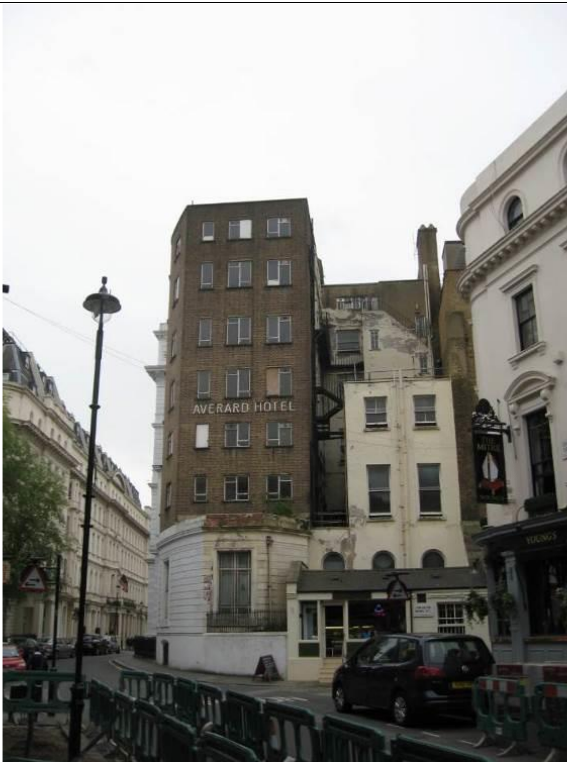
Rear (Craven Terrace) View
